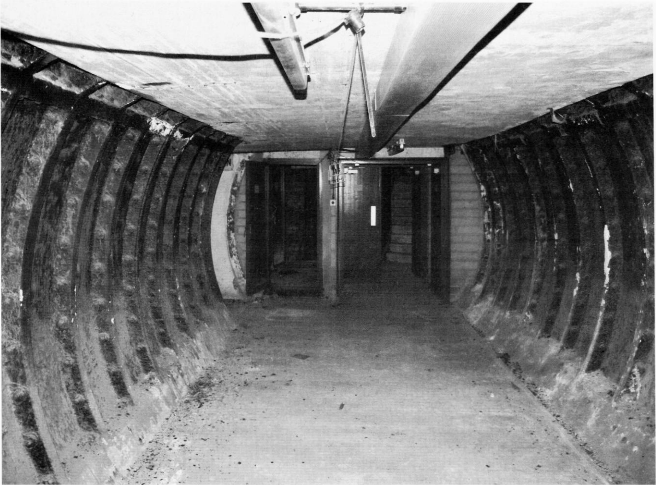
Looking back towards the spiral staircases in the crossover
